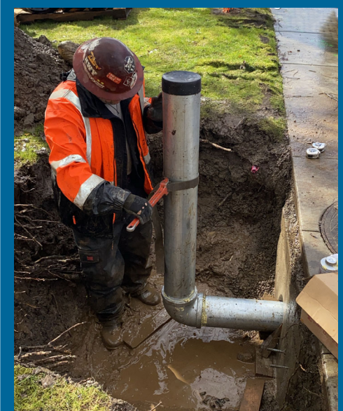
Emery crews install discharge piping.
