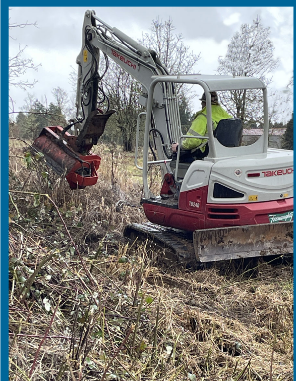
Emery crews clear brush at discharge site.
