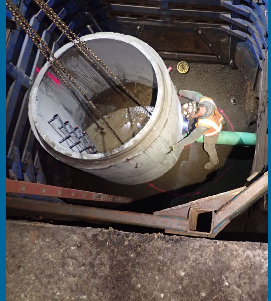
Oldcastle precast vault installation.
