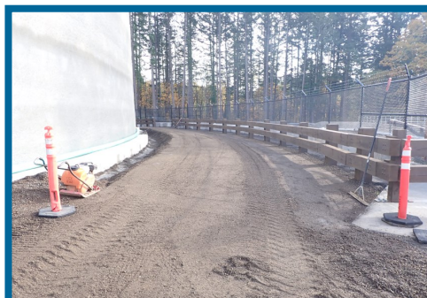
Site grading on the south and southeast side of the reservoir
