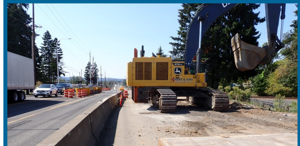
Bore pit excavation
