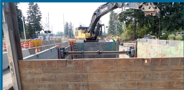
Bore pit at railroad tracks
