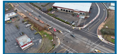
PLM_4.1: Aerial view of construction site
