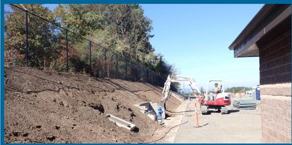
Project site south slope landscaping
