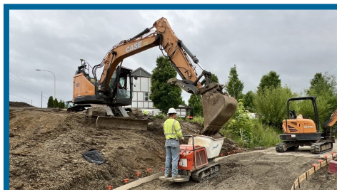
PLW_2.1: Preparing subbase for sidewalk placement
