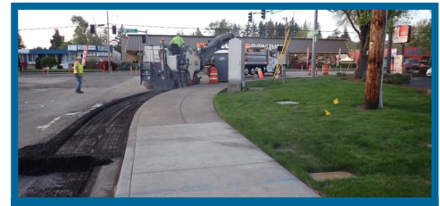
MPE_1.1: Grinding in preparation for street paving
