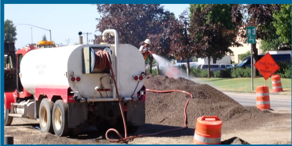
Adding water to the crushed rock
