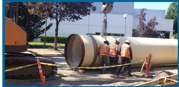
Crew rigging up the pipe for installation in the trench
