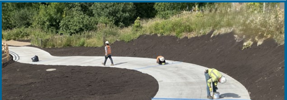
Installing expansion joint filler on new concrete trail in OWINP
