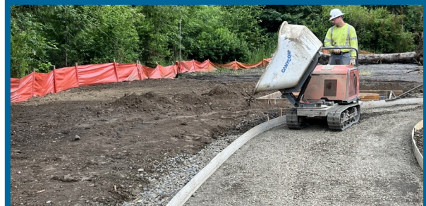
Placing drain rock at the edge of a sidewalk alignment
