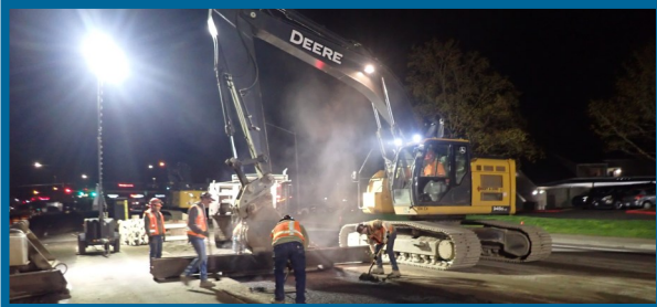
Paving 48-inch pipe trench on Scholls Ferry Rd
