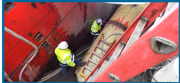
Magnetic particle inspection weld testing of 48-inch pipeline
