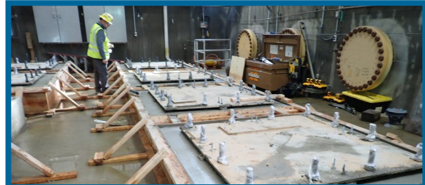
Freshly poured concrete for the Raw Water Facility pump bases
