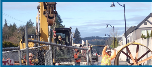
Preparing for tie-in between PLM_4.1 and PLM_4.4
