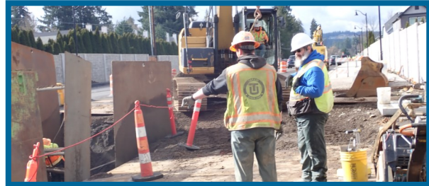
Backfilling after the connection between PLM_4.1 and PLM_4.4
