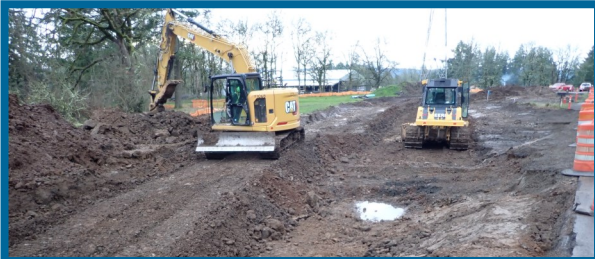
Topsoil replacement on easement adjacent to Koehler Road
