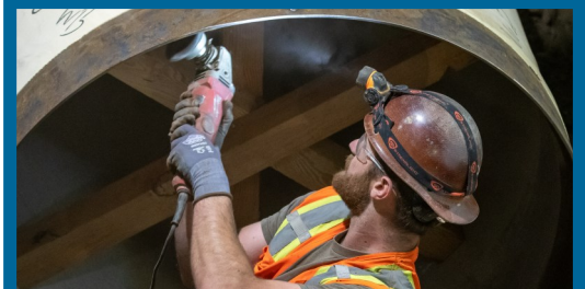
MPE_1.3: Contractor preparing pipe end for welding during night work
