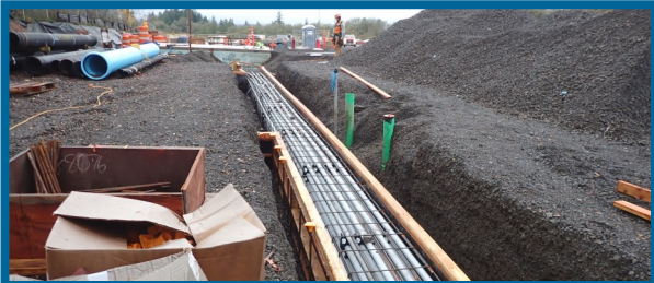
Electrical duct bank encasements
