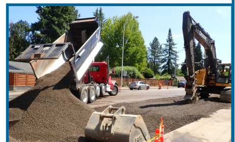
Removing shoring and backfilling at MPE_1.2
