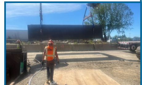
Placing flow meter vault pre-cast wall at MPE_1.1
