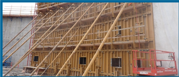
Formwork for prestressed concrete tank wall at the clearwell
