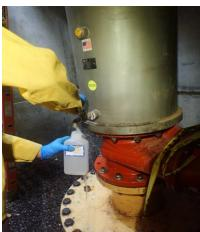
After pipe installation, the pipes are flushed, cleaned, and disinfected, and the water quality is tested. All this testing ensures the pipes are ready to deliver clean and
