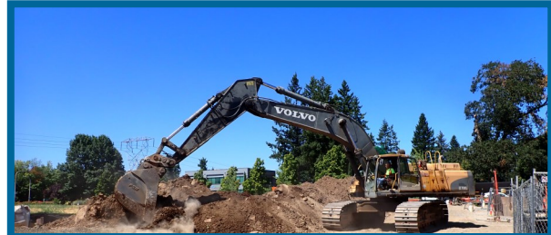
Stockpiling soil at the tunnel staging area near Wilsonville Road
