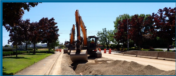
Backfilling a fiber optic conduit trench on 95th Avenue
