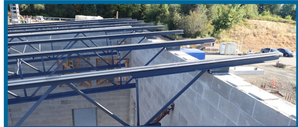
Upper site electrical building roof joist system
