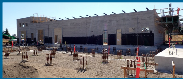
Upper site electrical building with lower one-third air barrier membrane applied
