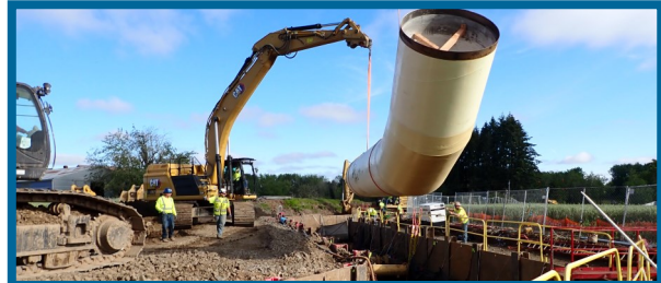
66-inch waterline installation north of Farmington Road
