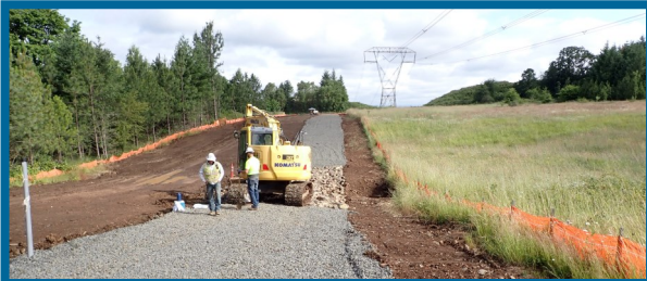
Permanent access road installation north of Greenslope Road
