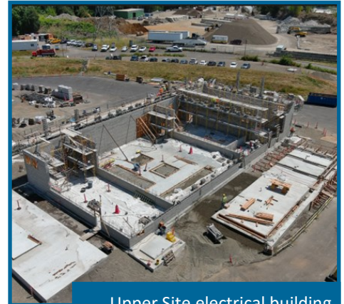
Upper Site electrical building south and west wall final CMU construction
