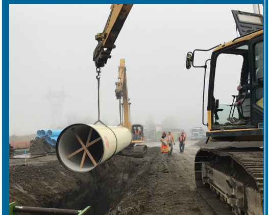
Northwest Pipe being installed.
