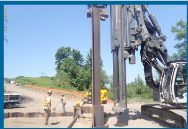
North shaft sheet pile install at Chicken Creek
