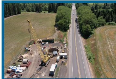
Receiving shaft at Tualatin River crossing
