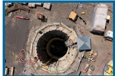
Overhead view of receiving shaft at Tualatin River crossing
