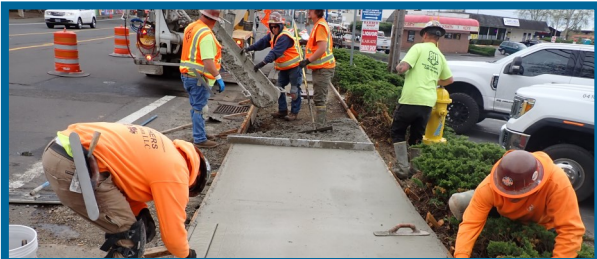
Crew pouring and finishing sidewalk along Scholls Ferry Road
