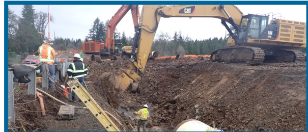
Trench excavation and slope cleaning along Grabhorn Road
