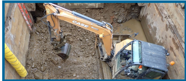
Contractor excavating the jacking shaft after slide rail shoring was installed
