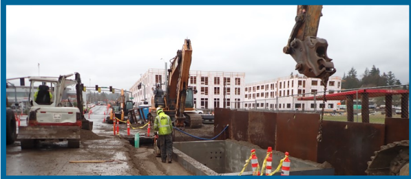
Backfilling and compaction around perimeter of flow-meter vault
