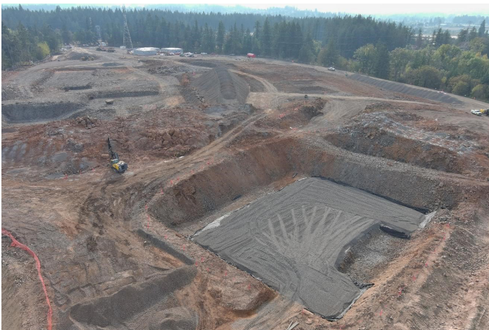
Equalization basin area subgrade
