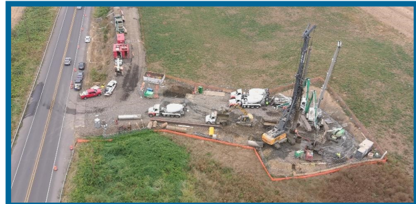
South Shaft Secant Pile Installation
