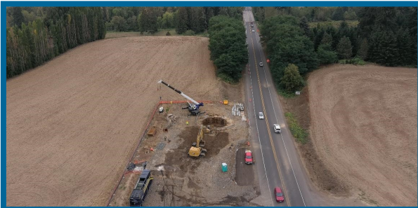
Excavation of North Tunnel Shaft
