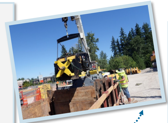
PLM_4.1: Lowering boring machine motor into launch pit
