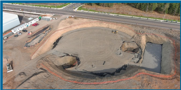
Water Treatment Plant Clearwell Area
