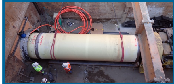
Installing 66" carrier pipe into a 84" casing.
