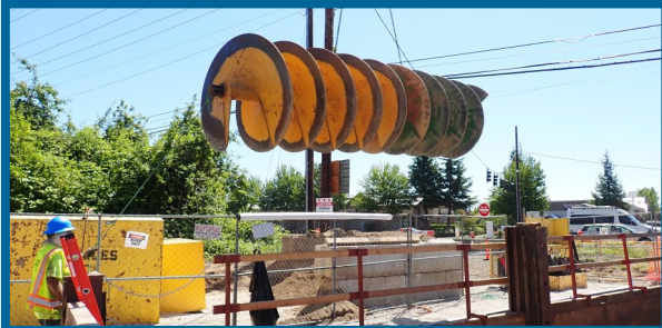
Lowering an auger into the launch pit.
