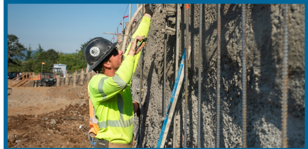
Iron worker installing rebar at Soil Nail Retaining Wall.
