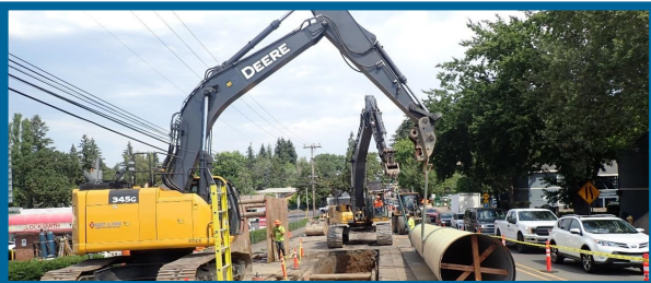
Installation of 48-inch waterline on Scholls Ferry Rd. near Hall Blvd.
