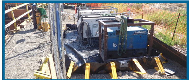
Dewatering pumps operating at Drive #1.
