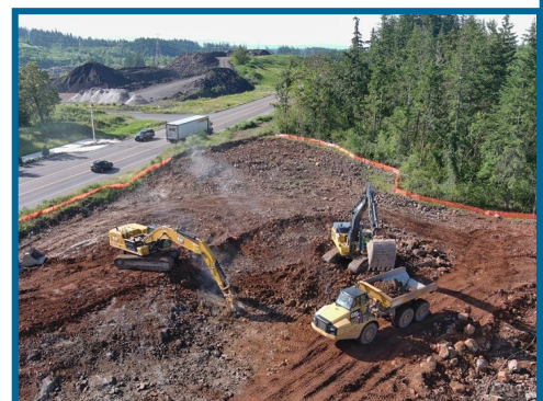
EXCAVATING AREA 35 CLEARWELL, AREA 53 PUMP STATION, AND AREA 54 SURGE MITIGATION
