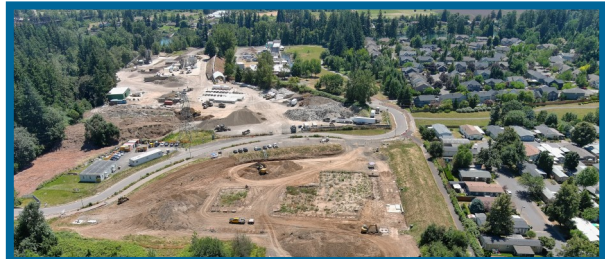
Upper site grading to final subgrades and excess soil haul-off
