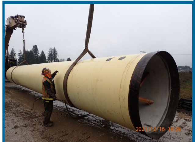
Pipe installation for PLW_1.3
