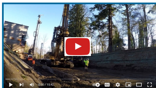
WIF Commission riverbank stabilization tour
