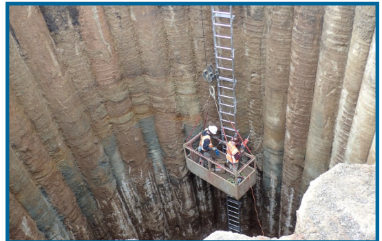
PLM_5.1 beginning of trenchless bore in jacking pit
