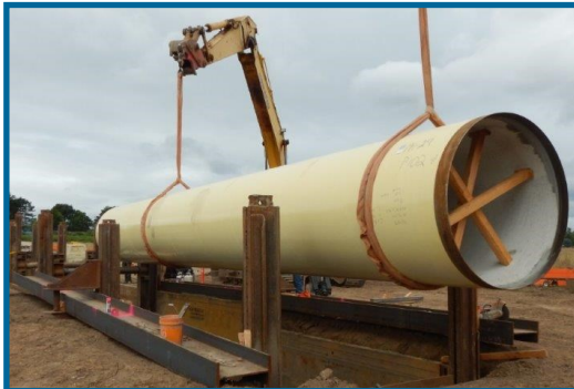
PLM_5.2 pipe installation "fly in"
