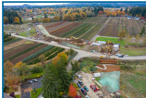
PLM_1.1 final construction and restoration
