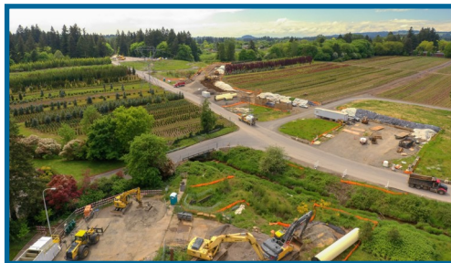
PLM_1.1 construction site looking southwest
