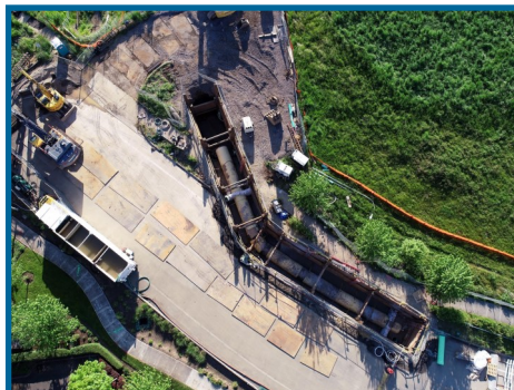
PLM_1.1 pipeline installation at Kinsman Rd.
