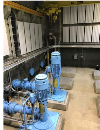
Existing WRWTP pump station
