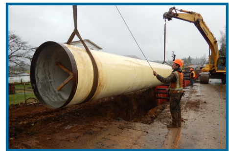
Installation of pipe for Scholls Area Pipeline Project (Phase 2)
