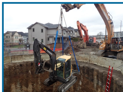
Excavation of jacking pit for Scholls Area Pipeline Project (Phase 1)
