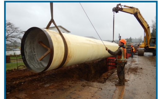
Installation of pipe for Scholls Area Pipeline Project (Phase 2)
