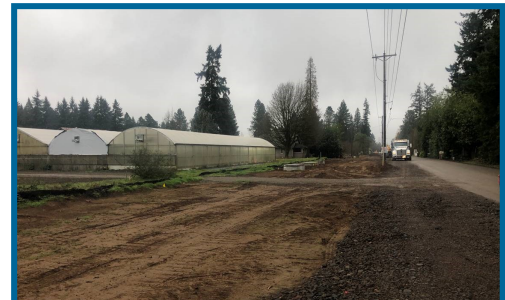
Wilsonville Area Pipeline Project Phase 2 construction
