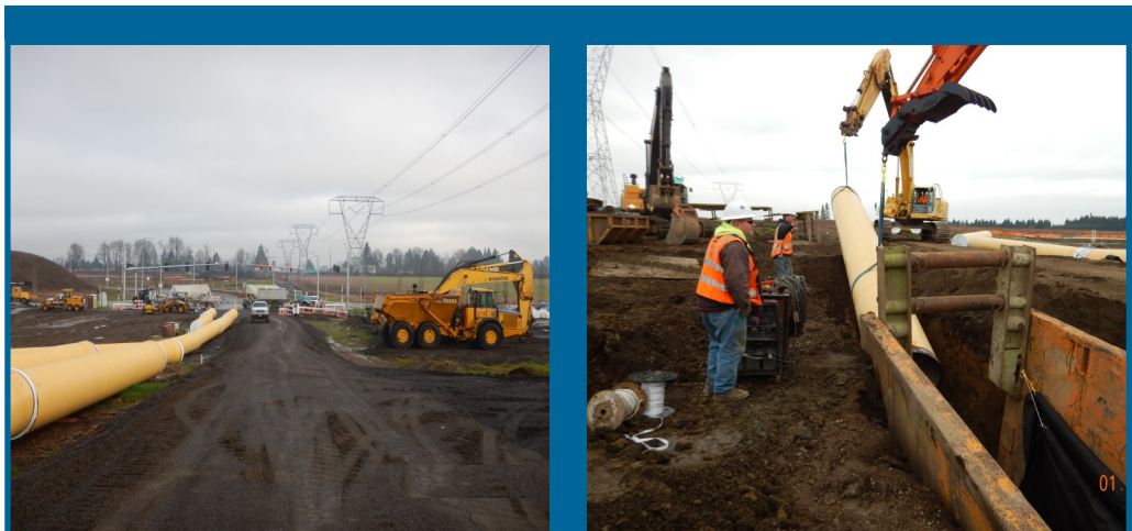
Installation of pipe at the South Hillsboro Area Pipeline Project
