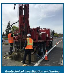
tion consists of drilling operations and collecting soil samples from boreholes at several depths and different locations along the alignment. The soil samples and rock cores obtained during site exploration and drilling are sent to a laboratory for testing to identify soil characteristics, including moisture content, density, permeability, shear and compression strength, corrosion properties (pH), etc. To date, more than 280 borings have been completed.
