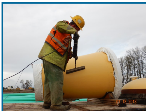
Testing pipe near TV Hwy for South Hillsboro Area Pipeline Project
