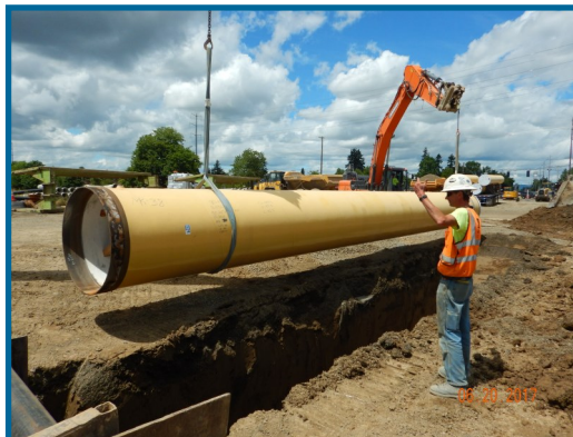
South Hillsboro Area Pipeline Project pipe installation
