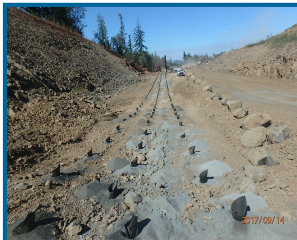
McCallum Rock Drilling of Salem drilled thousands of holes for the 124th Avenue Project to support recent rock blasting for construction. (video)
