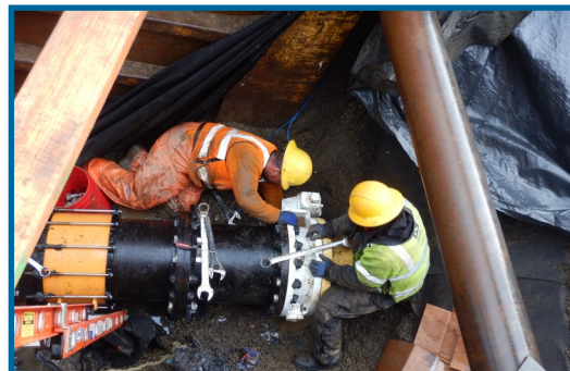
Construction work at South Hillsboro Project
