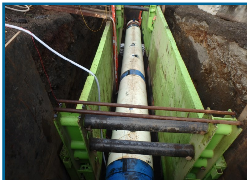
Installation of waterline for 124th Ave. Project
