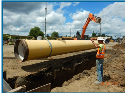
South Hillsboro Area Pipeline Project 48-inch diameter pipe installation
