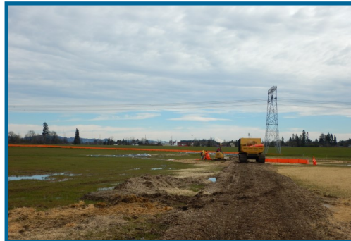
Installation of environmental control measures along South Hillsboro area
