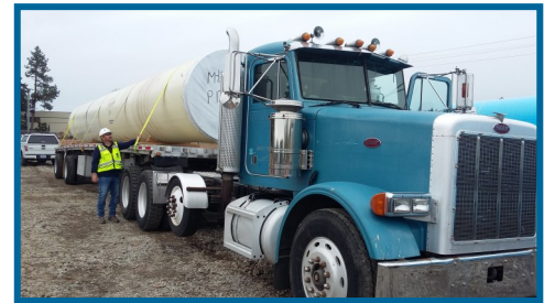
First piece of pipe for Willamette Water Supply installed October 11, 2016
