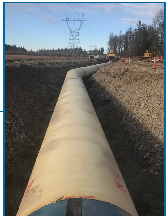
Kinsman Road Partnership Project pipeline looking north on future Kinsman
