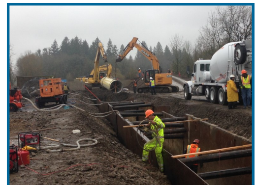
Installing 66-inch diameter pipe on Kinsman Rd.
